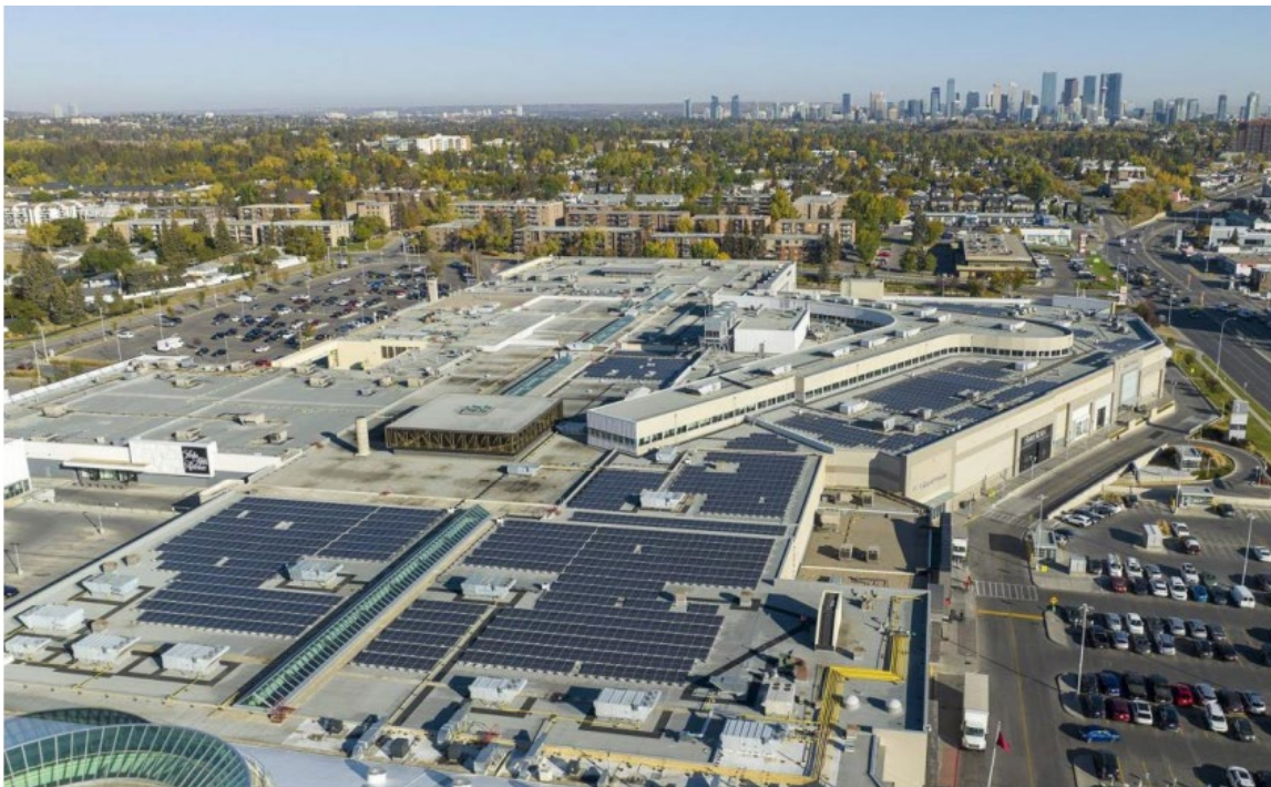
Aerial view of CF Chinook Centre solar installation
