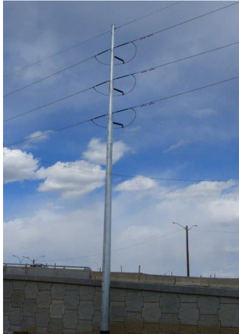
Proposed single circuit dead-end monopole
