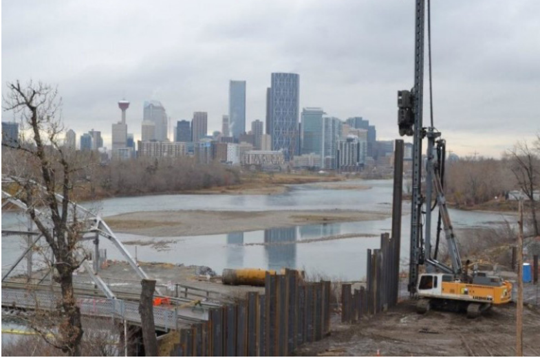
Example of Sheet Pile Wall construction
