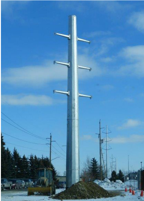
Proposed double circuit dead-end monopole
