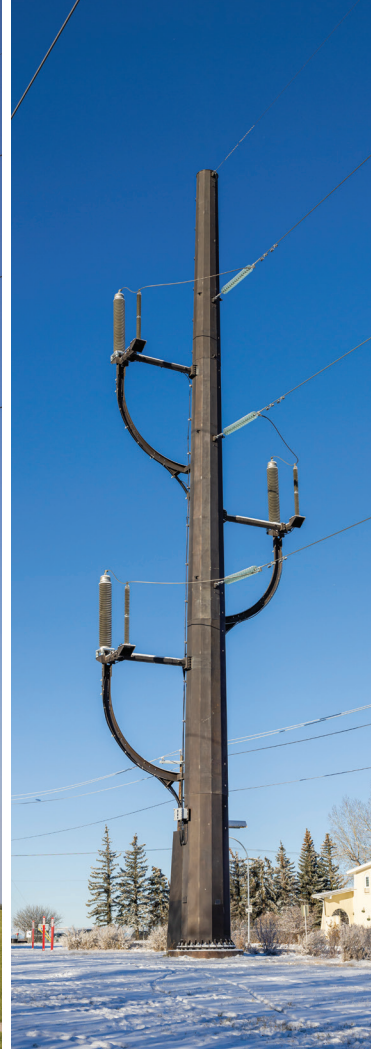
Example of Riser Structure (Typically a Self-Supporting Steel Monopole)
