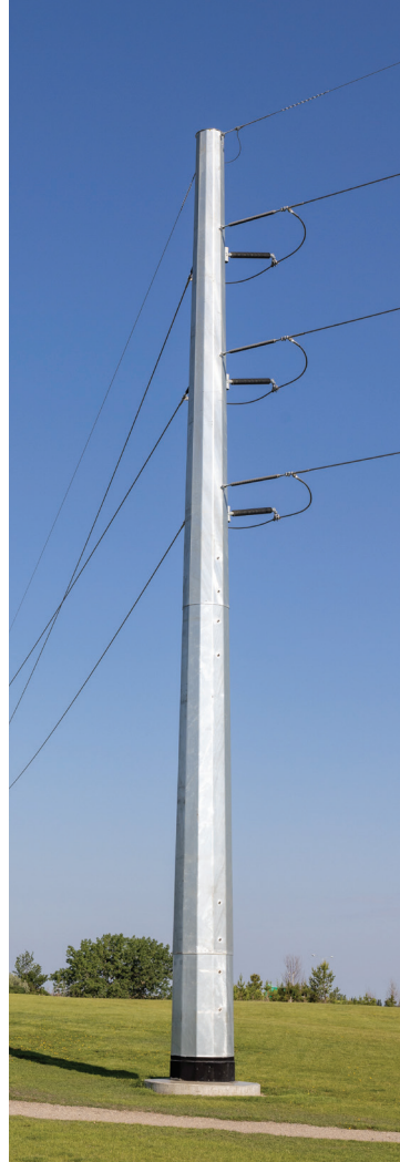
Example of Self-Supporting Steel Monopole
